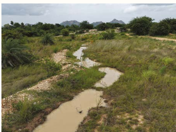
▲ Contour trenches holding moisture for longer periods, indicating improved infiltration across the site.
