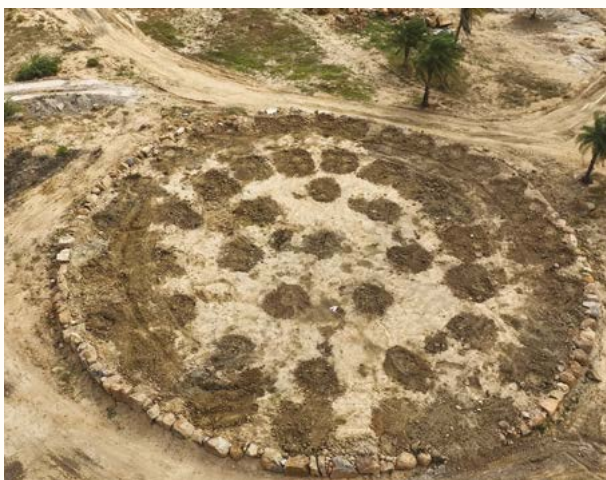
▲ Elevated mound built using local rock and mud to support water-loving plants, creating seasonal refuges for birds in the middle of the inundated area
