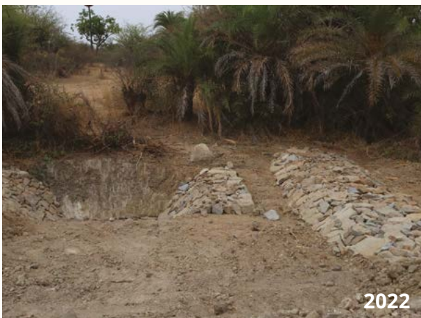
▲ Dug-out ponds and gully plugs slowing runoff and allowing water to spread and soak into the soil along drainage lines.
