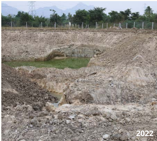
▲ Seepage well, gravity-fed by aquifer recharge from upstream watershed structures and functioning as a water supply point for site operations.
