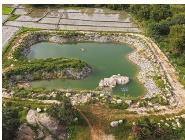
▲ Seepage well retaining water into the dry season, with a holding capacity of 6.5 Million L.
