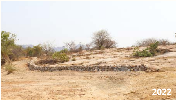
▲ Pebble and stone bunds stabilising slopes, reducing erosion, and retaining moisture at the surface.
