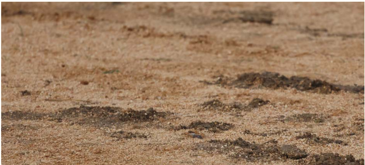
▲ Compacted soils and exposed subsoil on sloped areas within the Veltoor site.
