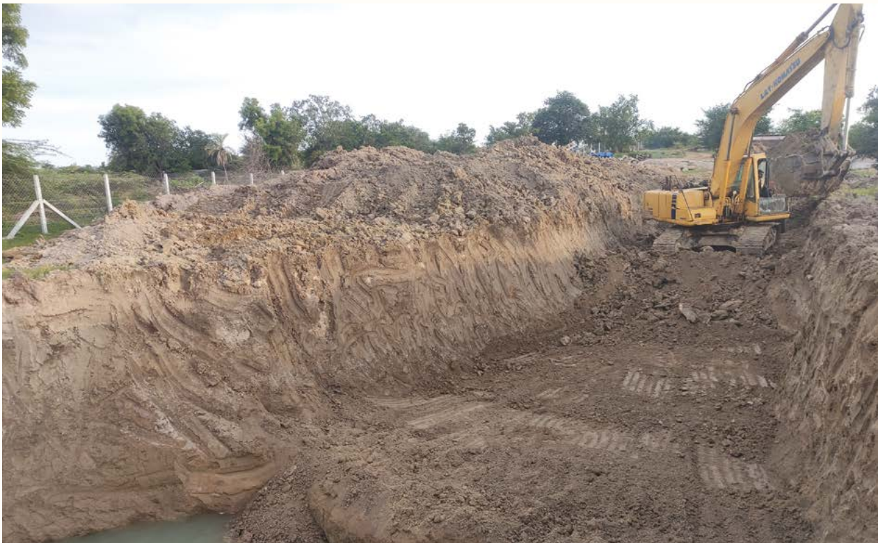
▲ Building a Seepage Well at the site's lowest point, where gravity passively gathers aquifer water recharged by upstream watershed structures.
