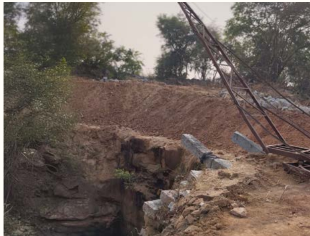
▲ Revival of an old well at Veltoor using local materials and traditional methods.
